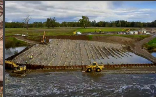
South Dubbo Weir
