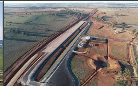
Parkes Logistic Terminal
